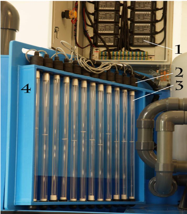
**Fig. 5: 12 x UV-C lamps with 20 watts each**
